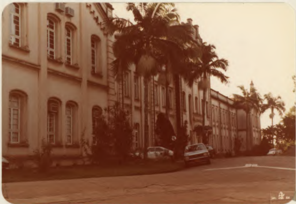
4) Prédio Principal ( Fundos )
