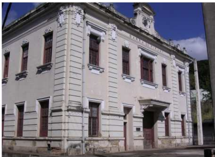
fachada principal e cunhal
