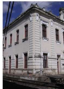
fachada principal e cunhal
